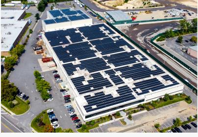
of LG 405 and LG 400 panels, TerraGen solar racking, and Solectria inverters.
