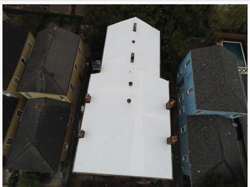
Central City historic home with WrapRoof installed
