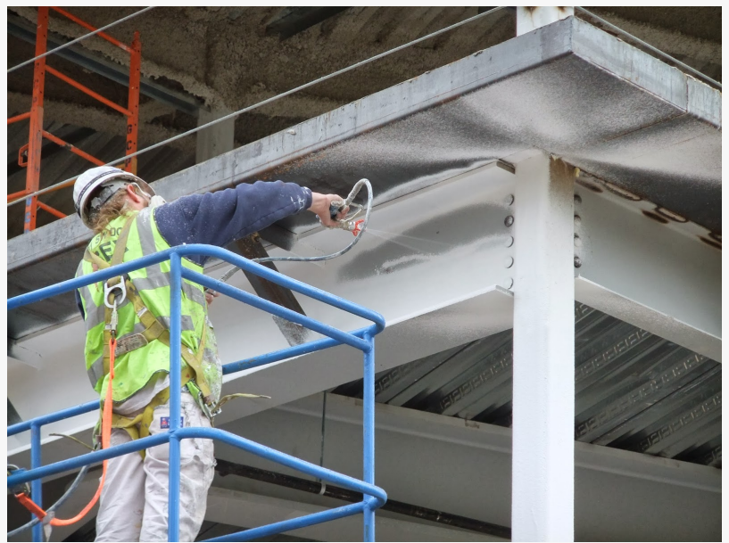
Fire Protection Coating Market
