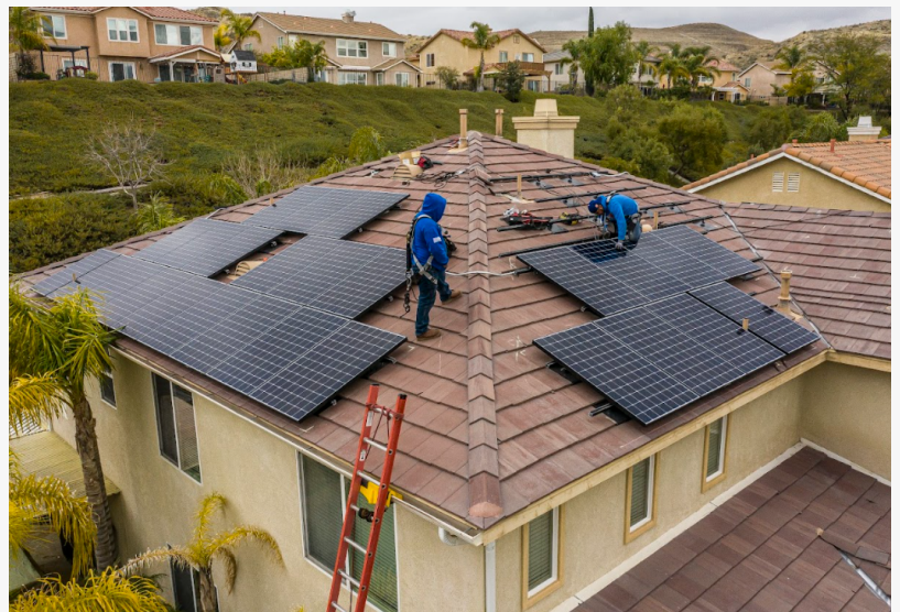
Cervus Residential Solar Installation
