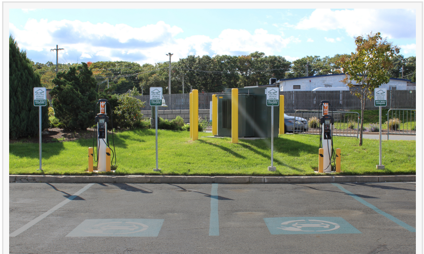
Bally's Twin River Level 2 Chargers Installed by Inovis Energy
