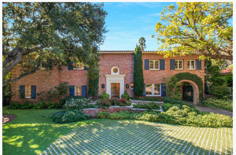
Bridges to Recovery, Beverly Hills—Maple Drive
