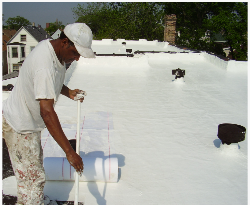
Energy-Efficient Roof Coating Application
