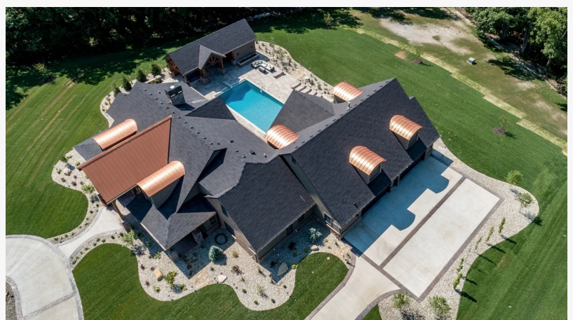
Arizona Home Inspection of Residential Roofing
