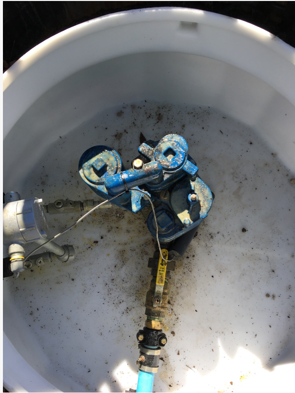
Same ethanol pump, 359 days later, shows no sign of corrosion
