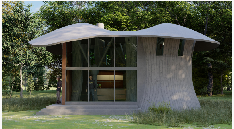
3d printed sustainable concrete Canopy™ House by Madco3d uses two types of 3d printing to achieve.
