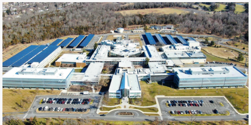
ECS energy Elnik Installation
