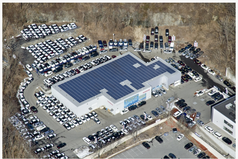
ECS energy Central Ave Nissan Installation
