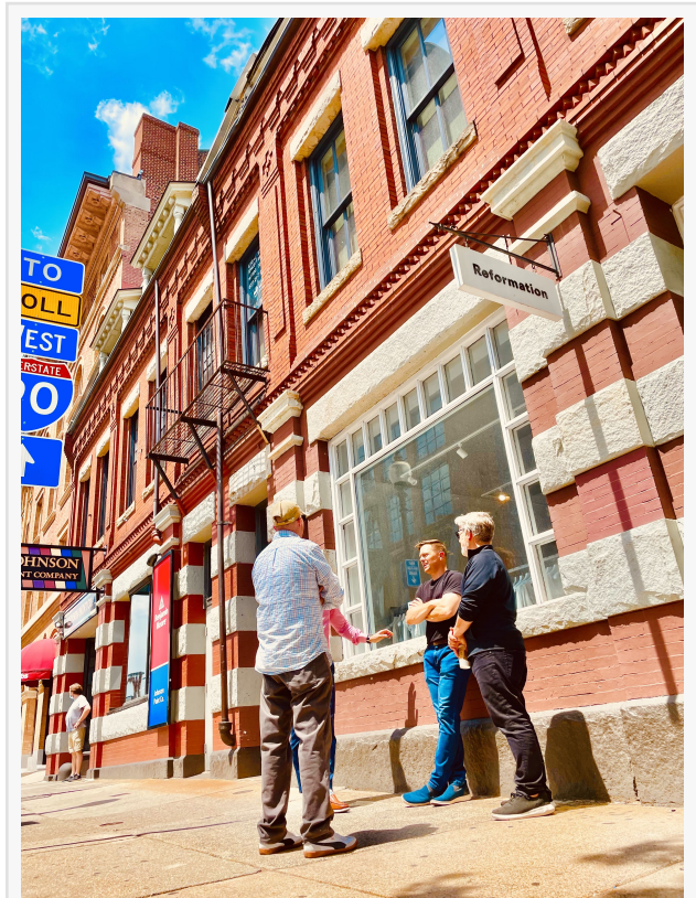
FableVision Studios' new home, a multi-story brownstone with roof deck on Boston's iconic Newbury Street
