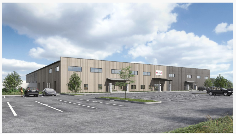
Satellite Industries New Deodorizer Manufacturing Facility in Cedar Park
