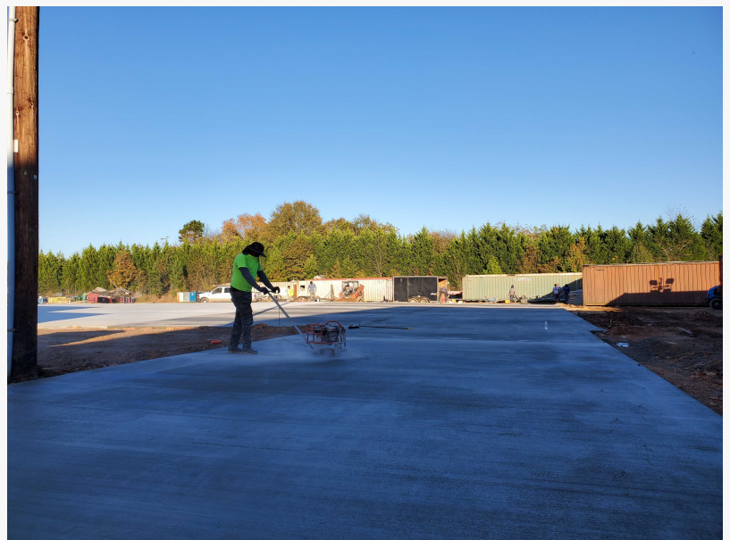
Concrete poured for new interim inventory location.
