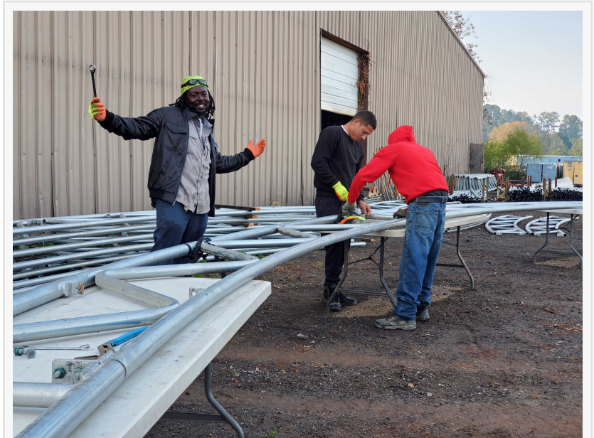
GE&S Staff starting to assemble new interim inventory structure.
