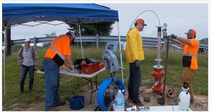
Electro Scan's Robotic TRIDENT Probe Is Easily Inserted into Common Hydrants, Navigating Multiple 90-Degree Bends For Up to 400ft (120m) Pipe Surveys.
