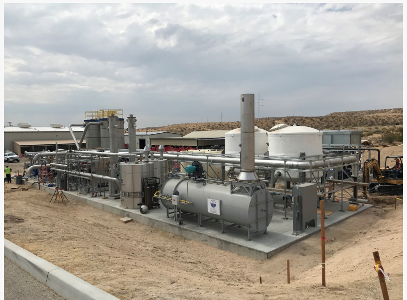
Ship & Shore System comprised of Thermal Oxidizer, Scrubber, and a series of Lead Lag Vessels
