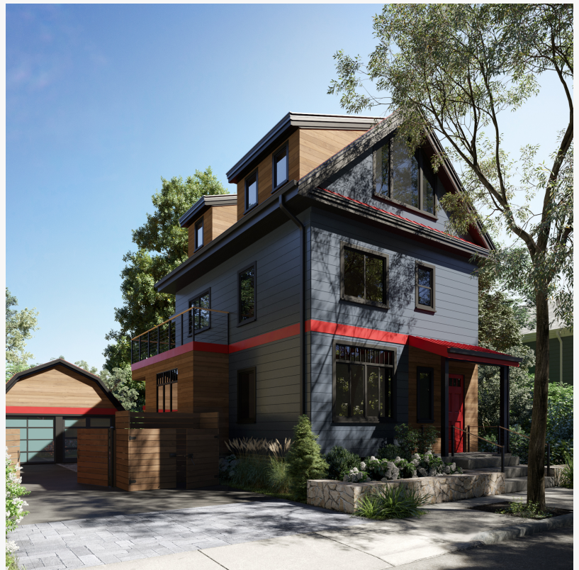
Photo-Realistic Rendering of a Passive House Currently Under Construction
