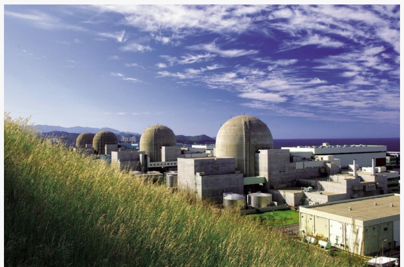
The Hanul power plant in South Korea, which uses an Australian Technofast CamNut® system not only to increase operational safety, but also to boost generation uptime
