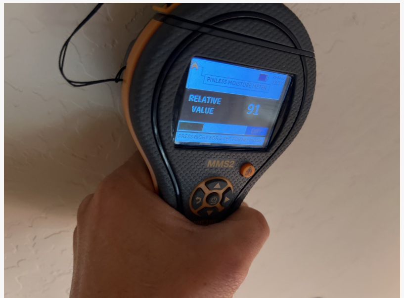
Using a moisture meter to find hidden moisture inside walls.
