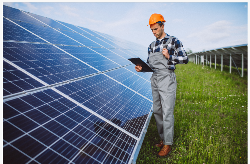
Solar Panels Power Monitoring & Cleaning
