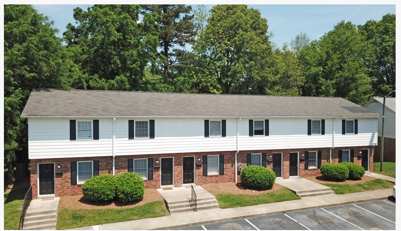
Four Seasons Villas (96 Units)
