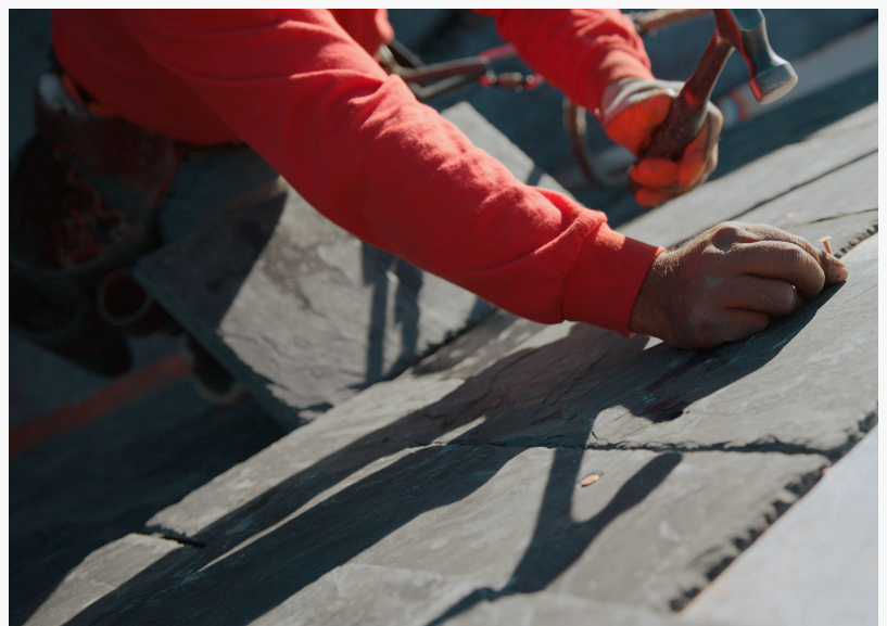
Guy Roofing installs a high-end slate roof.
