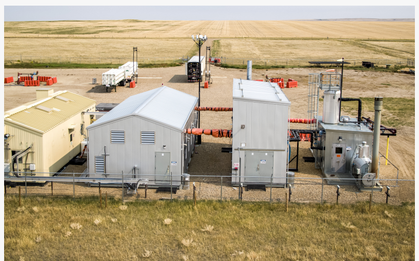
The helium well can process in excess of 6MMscfd of helium-bearing gas
