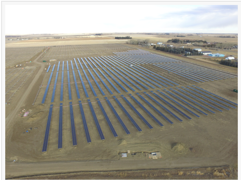
Brooks Solar II Site - picture provided by Elemental Energy Inc.
