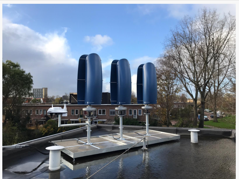
Flower Turbines Small Size Wind Tulip Installation
