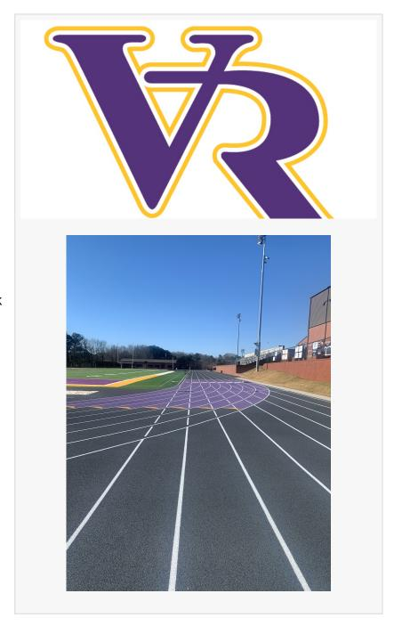
temperatures and feels like a natural surface with increased traction and footing for athletes. The track renovation included expanding the existing six-lanes to eight and the installation of new synthetic surfacing. The Rekortan BS synthetic track surface will endure higher wear and traffic along with providing enhanced force reduction for athletes.
