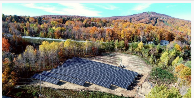
Bromley Mountain Ski Resort's new solar array mid-construction this fall
