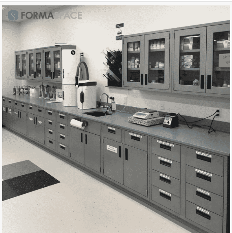
Shown above is a custom steel casework installation featuring a gray epoxy top and backsplash, black epoxy resin sink, faucet, epoxy pegboard drying rack, eyewash station, and a stainless steel drip tray.
