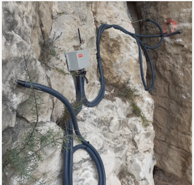
A Worldsensing wireless datalogger connected to a crack meter is used to monitor a rock cliff along the rail line from Lleida to La Pobla in Catalunya, Spain. From Ferrocarrils de la Generalitat de Catalunya (FGC)
