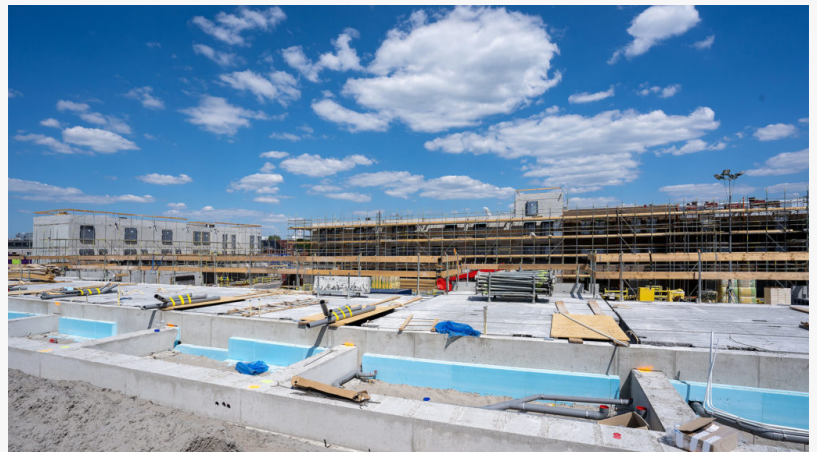
Boron in Construction Materials - Borates Today
