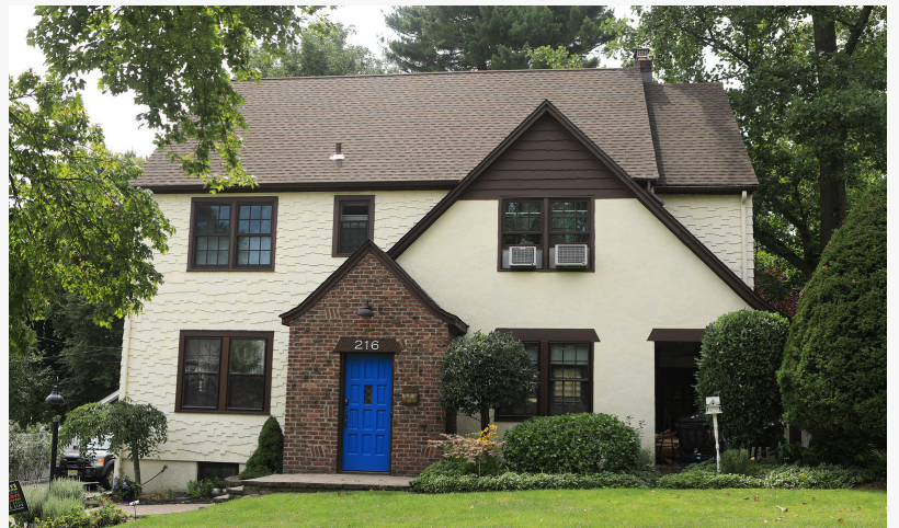
Gikas roofing services
