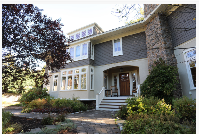
Gikas roof repair
