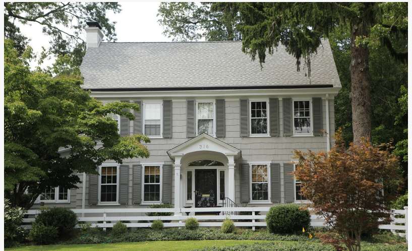
Gikas Roofing reconstruction: the subtle nuances of the roof project
