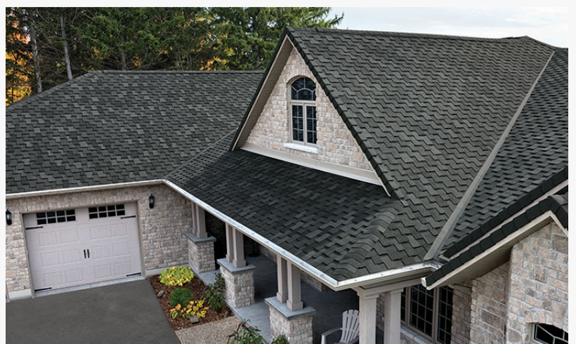
new roof installation
