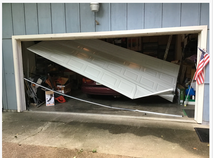
door off track repair
