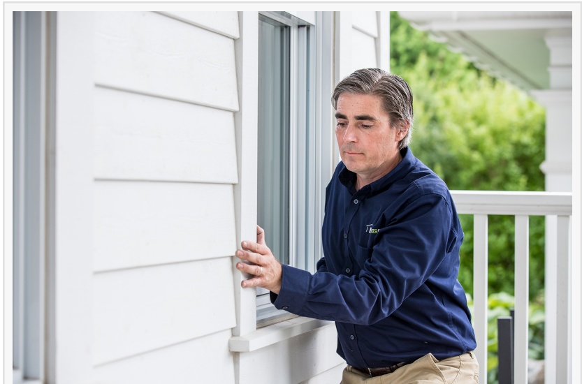
A Pillar To Post Home Inspector Checks a Window Frame for Leaks
