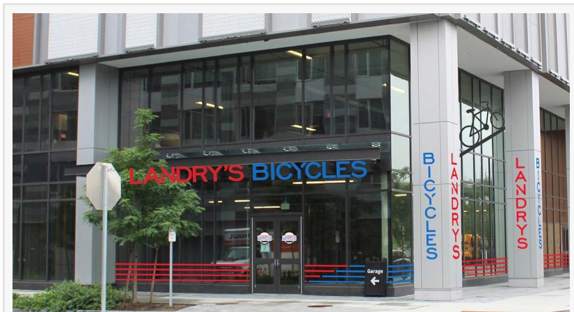
Preliminary rendering of Landry's new store location in Charlestown. The new store is expected to open early this year.
