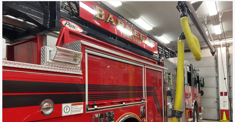
Barnegat Volunteer Fire Department installed A Fire Station Vehicle Exhaust Removal System
