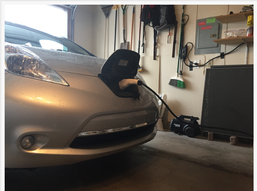
MySolar Home Car Charger Residential Solar Installation Jan. 2022 Contact Us at 505-705-1111
