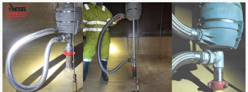
DieselCare Skimmer® fuel station installations in Scandinavia.
