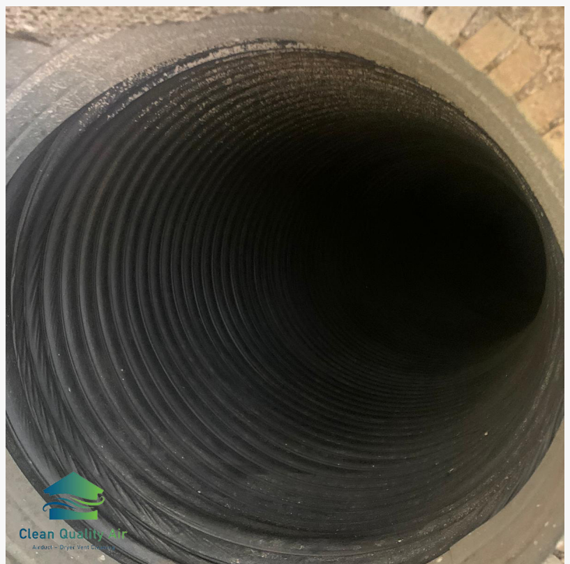
Comprehensive Air Duct Cleaning
