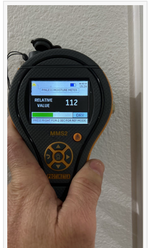
Avondale Moisture Meter of Water Damage
