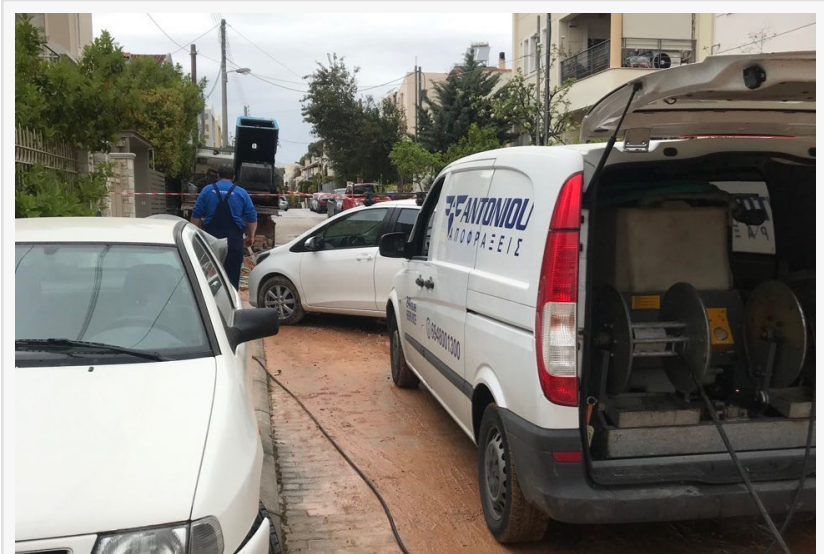
repair of a drain system
