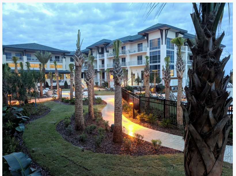
New addition tot he Embassy Suites Resort on St. Augustitne Beach complete in 2022.
