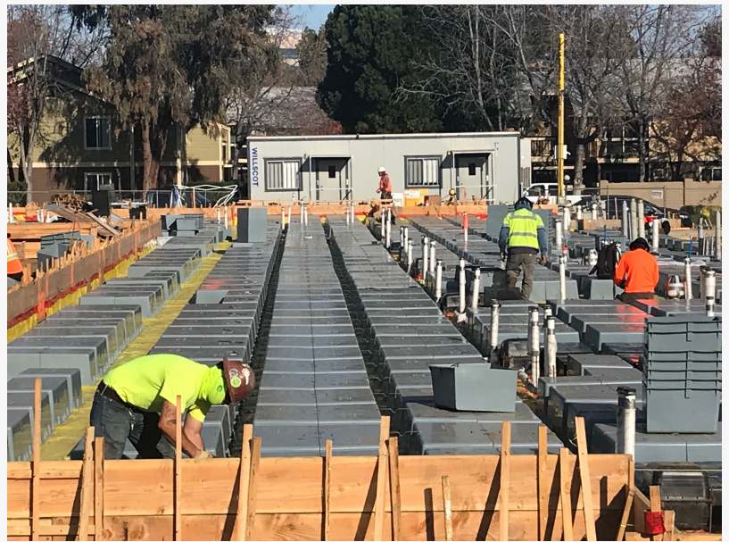
Wafflemat is installed quickly and easily with Waffleboxes and Connector Clips.
