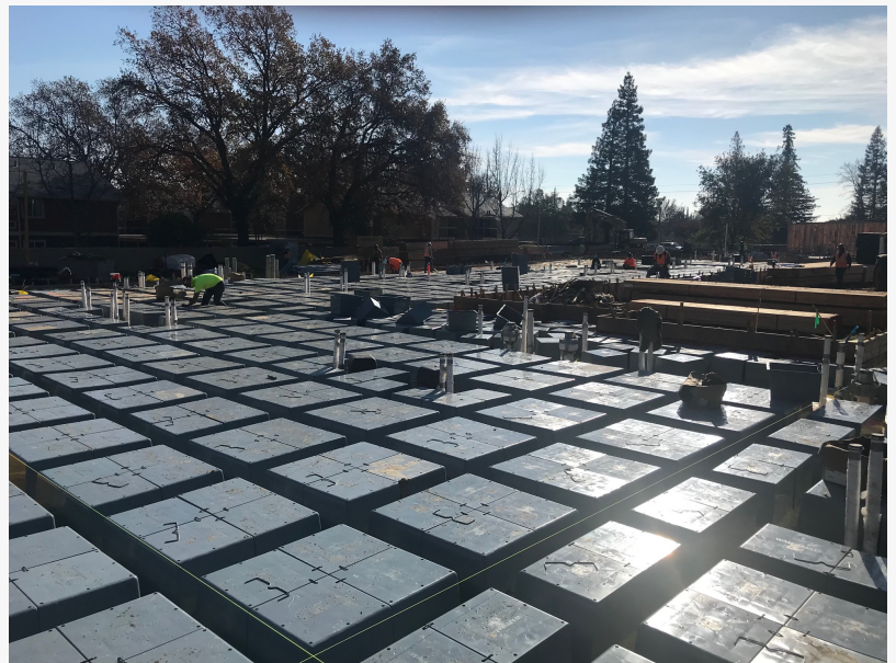
The Waffle Pod Slab Design allows for soils to expand and compress in the void forms, keeping the pressure from cracking the concrete.
