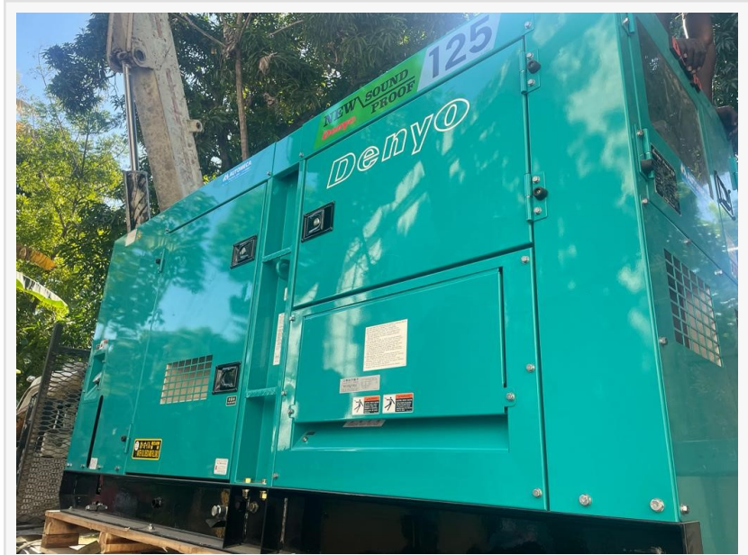
New generator allows Hopital Sainte Croix in Leogane Haiti to re-open following hijacking.
