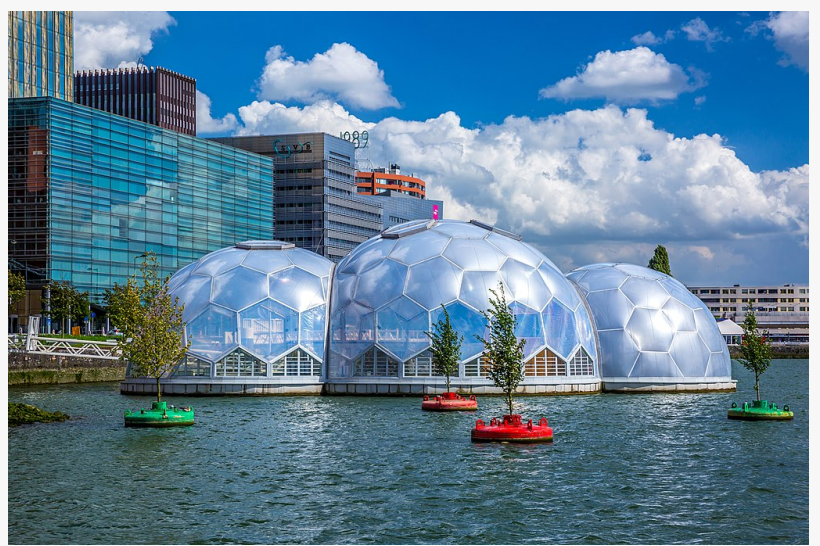
The Rotterdam Floating Pavilion in the Rijnhaven district.
