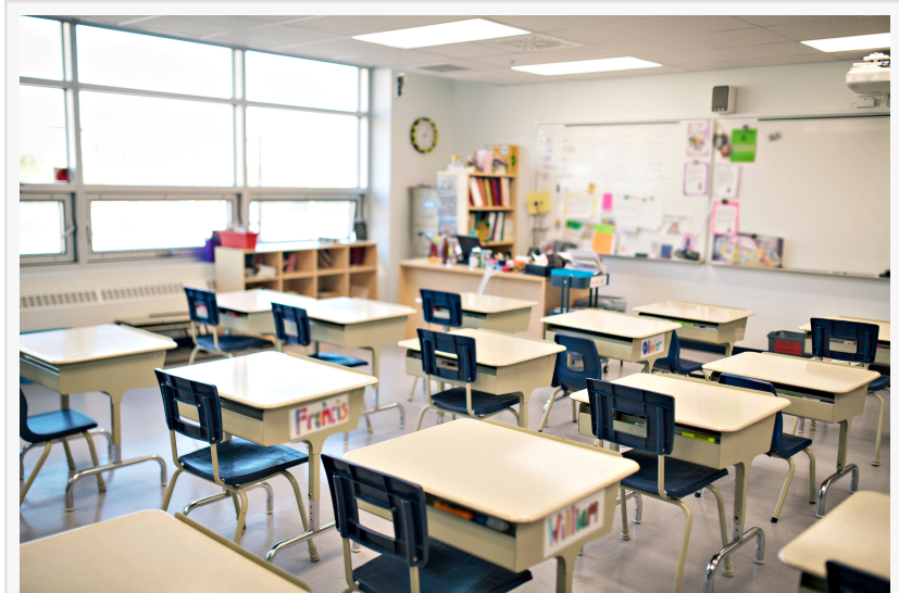
Delos School Air Purification System
