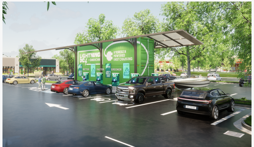
Charging Plaza Incorporating Hydrogen Technology
