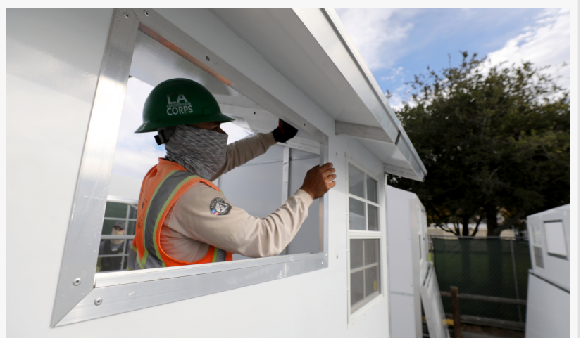
Assembling a Pallet Shelter.
