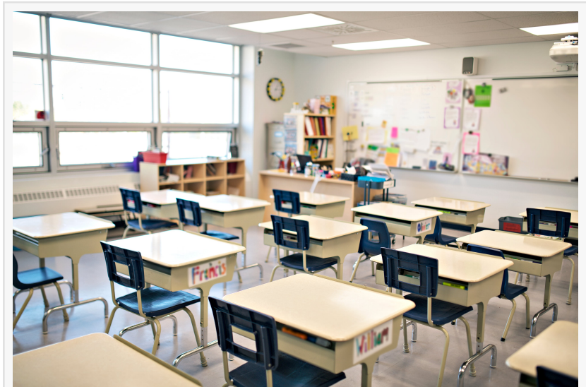
Delos School Air Purification System
