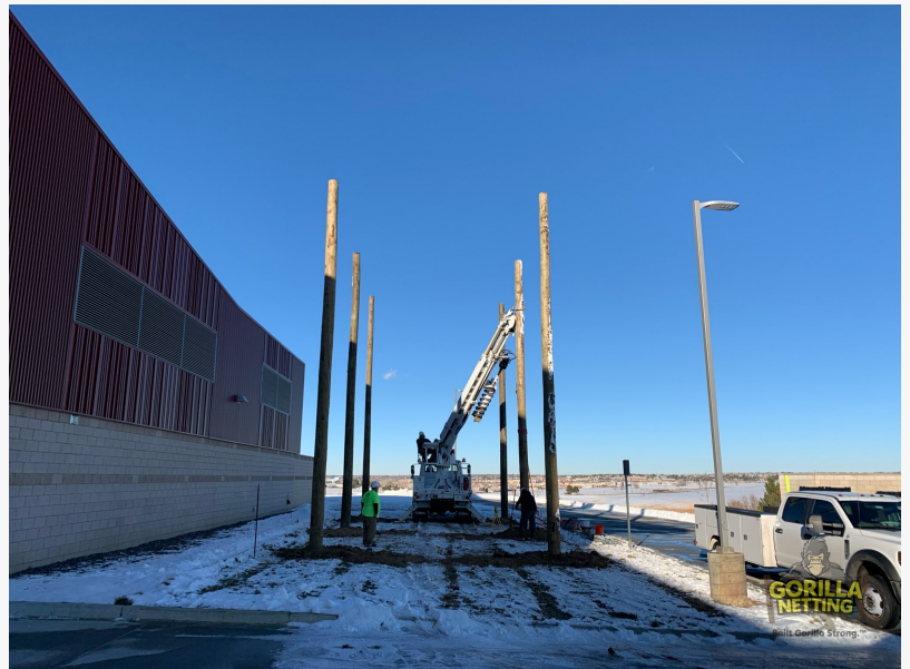
Gorilla Netting crew members install support poles for the drone enclosure being installed at CCIC
